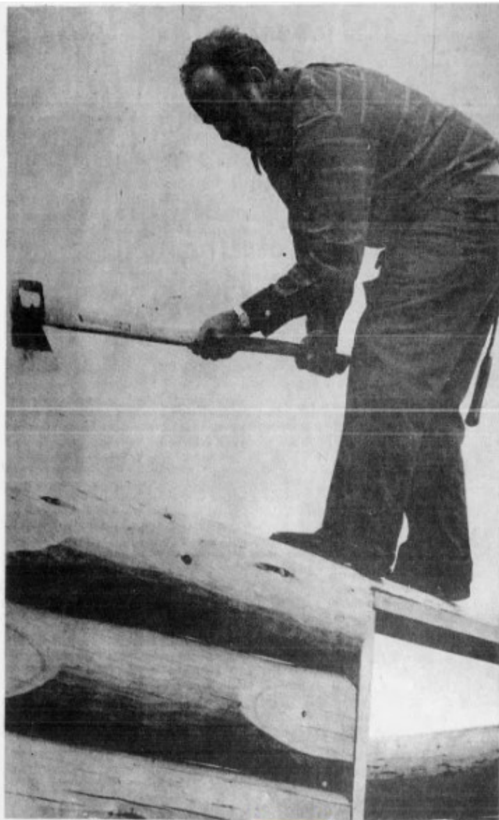
TOURIST BOOTH CONSTRUCTION — Don Olson wields an axe at the city chamber of commerce visitor information booth west of the city. The booth was scheduled to be opened in mid-June, but an end-of-month opening seems more realistic at this time. Work on the booth is strictly volunteer.
