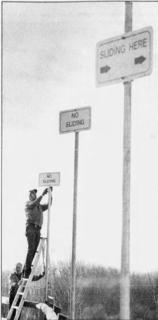
City facility maintenance workers Leslie Burrows (holding ladder) and Larry Crerar install signs at top of Suicide Hill.
