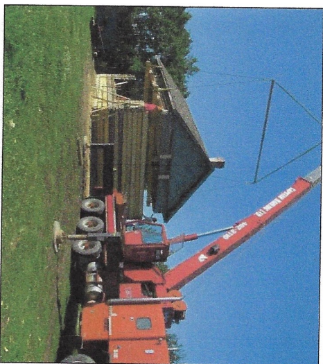
Top left: A crane removes the roof and top three logs of the Glen Leslie Church, 2013.
