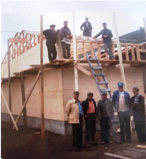
left building addition on Legion Hut.
